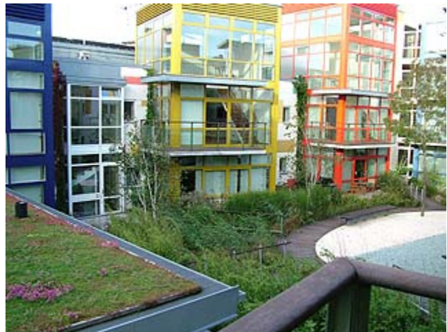
Photo courtesy of International Sustainable Solutions In Malmö, Sweden, this housing complex filters stormwater through green roofs and specialized landscapes.
