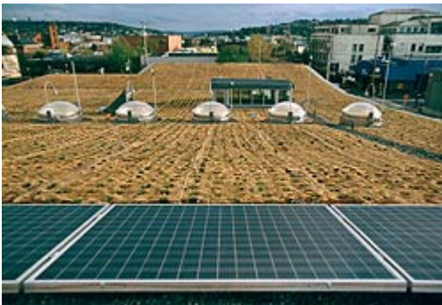
On the roof, solar panels (foreground), sod and weather instruments(background). (Nic Lehoux)
