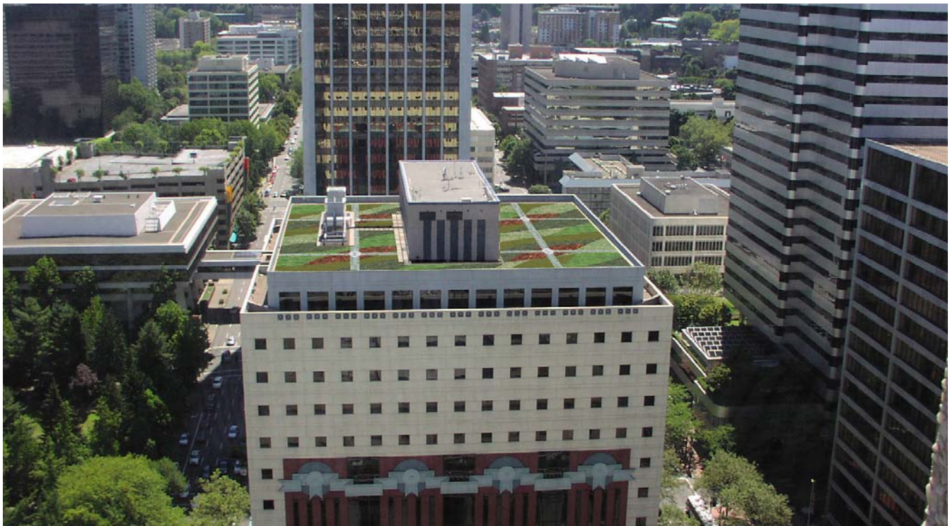
Proposed design for the Portland Building Green Roof – Graphic by Andrea Saven, Macdonald Environmental Planning
